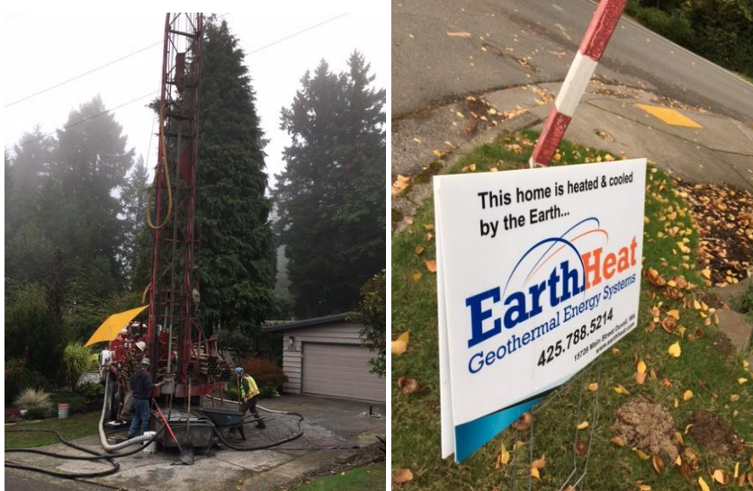
Drilling rig for a ground-source heat pump's circulating refrigerant lines.
